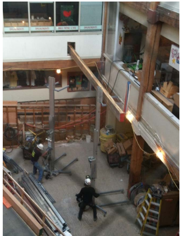
Loading Drag Struts for DeLaurenti
