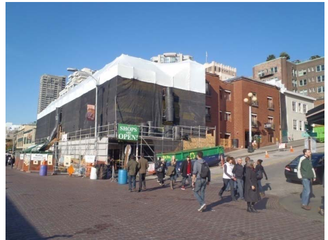
Stewart House Pike Scaffolding
