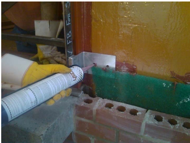
Installing Railing at Stewart House
