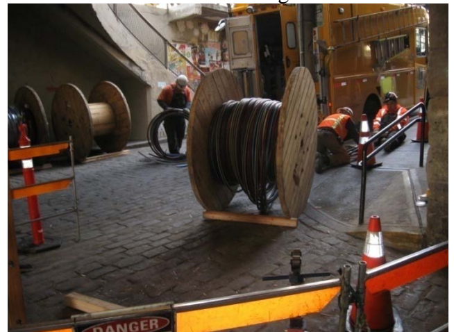
Electrical Wiring installation: Post Alley
