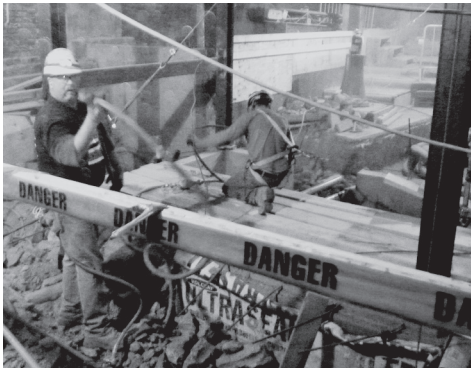
Above: Duct bank (underground electrical cables) demolition inside the Market Theatre.
