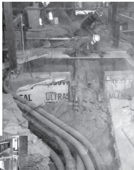
Left: Electrical wiring installation off of Post Alley.
