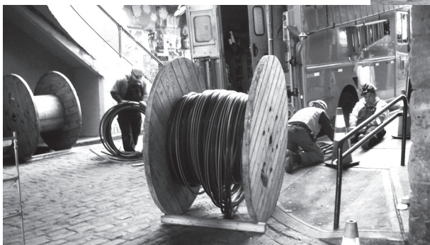
Left: Electrical wiring installation off of Post Alley.
