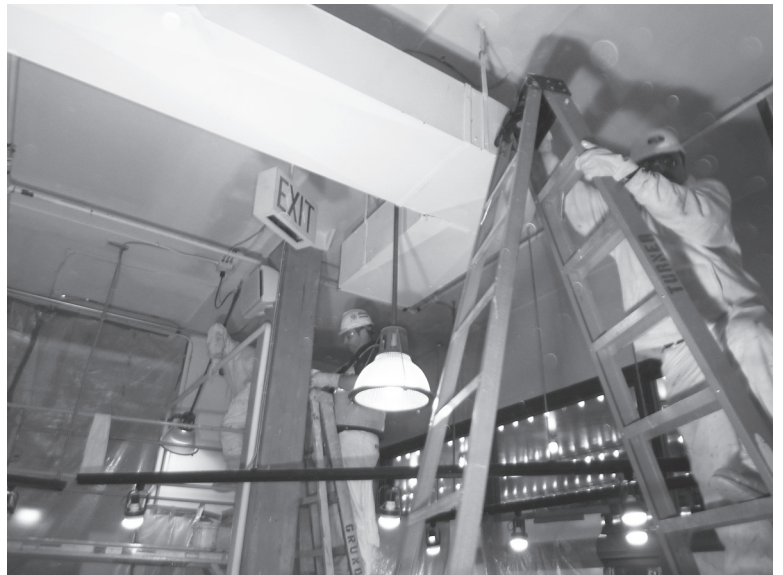
Above: Reinstalling ductwork inside DeLaurenti's.
