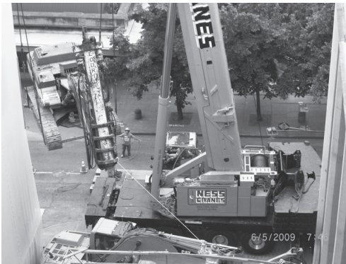
A crane that can lift 550 tons—only two this large exist on the West Coast!—was brought in to lift the Lodril (seen in the upper left) into place.
