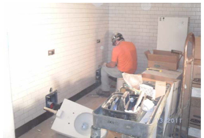
Toilet Install Women's Public Bathroom 602
