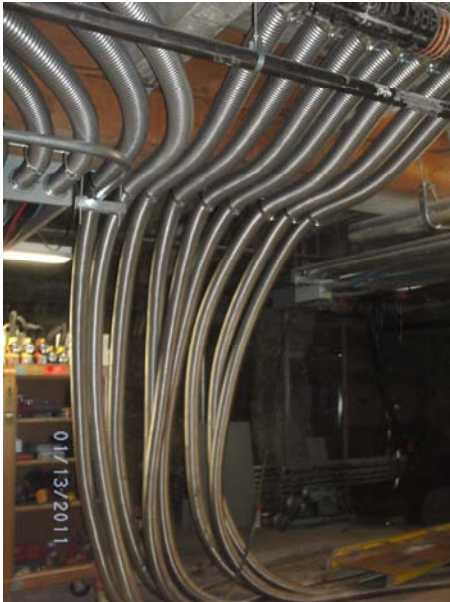
Piping in the Triangle Basement
