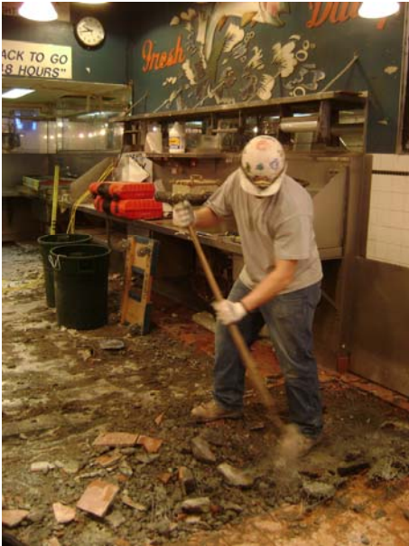
Chipping away the old tile floor at Pure Foods Fish
