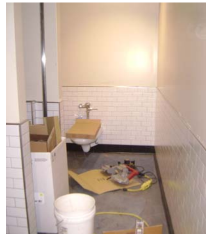
Tenant Bathroom 702 in the Corner Market
