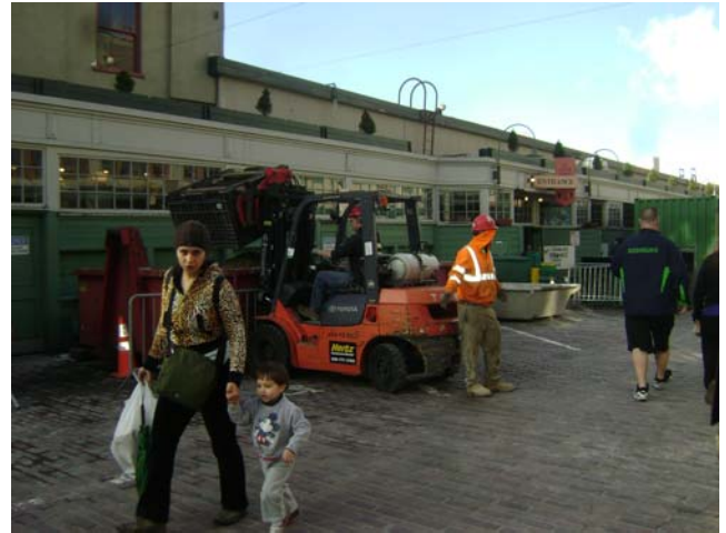
Dumping debris safely while keeping Pike Place open to pedestrian traffic
