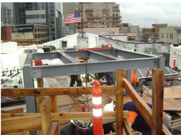
Top of the Elevator Shaft-Corner Market
