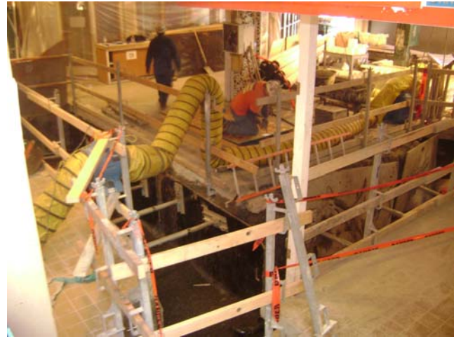
Main Plumbing Trench Sanitary Market
