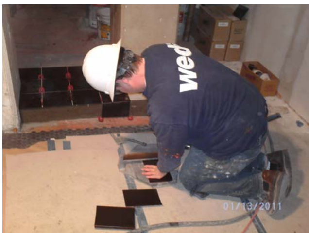
Tile cutting for the Public Bathrooms 602
