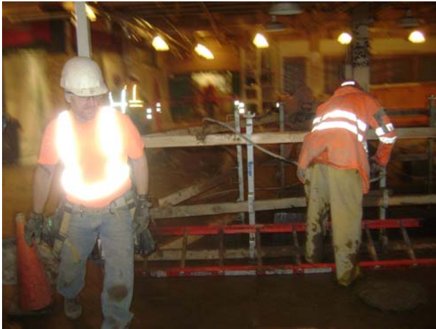
Main Plumbing Trench Sanitary Market
