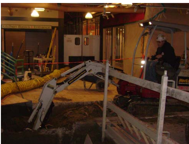
Excavation of the Sanitary Market Trench
