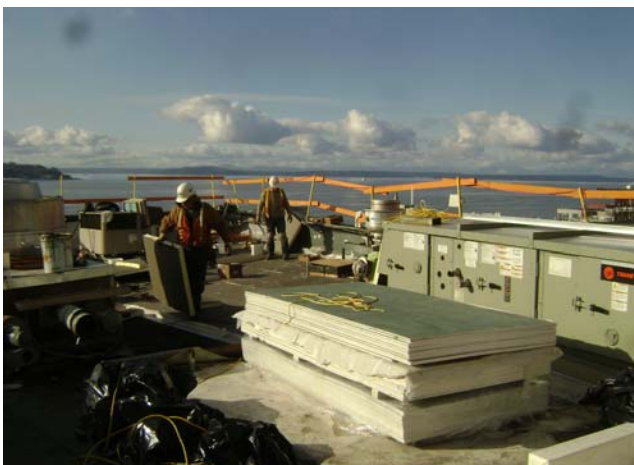
Corner Market Roofing
