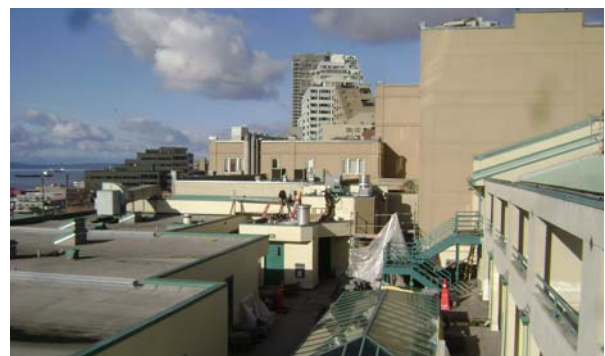
Stucco Work on North Shaft Sanitary Roof
