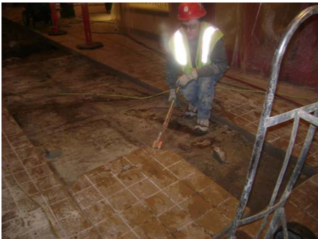
Main Plumbing Trench Sanitary Market
