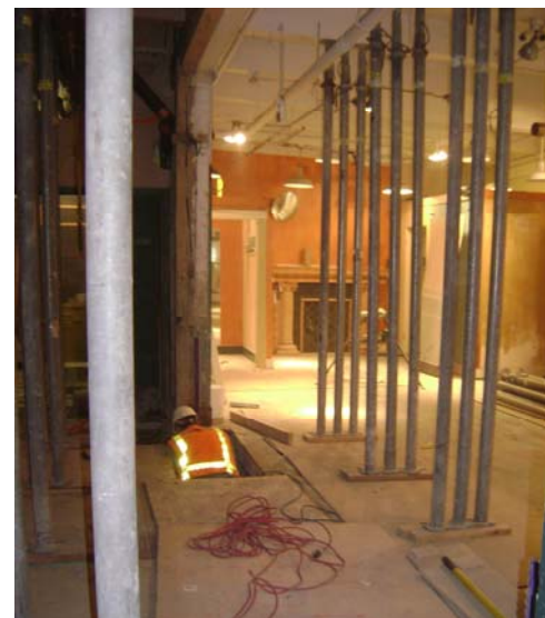
Shining Star Brace Frame, footing prep
