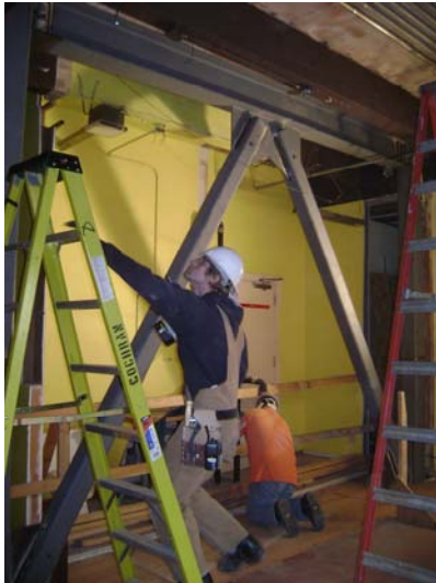
Electrical work in Bohemia; French Fry Brace Frame in the background
