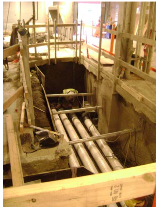
Condenser water piping installation in the Sanitary Market
