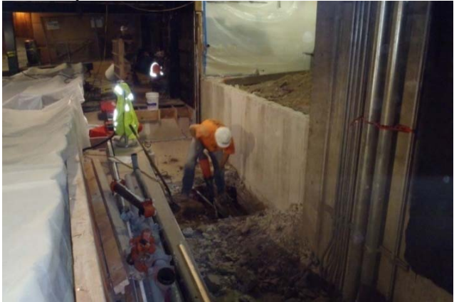
Economy Market Footing Excavation
