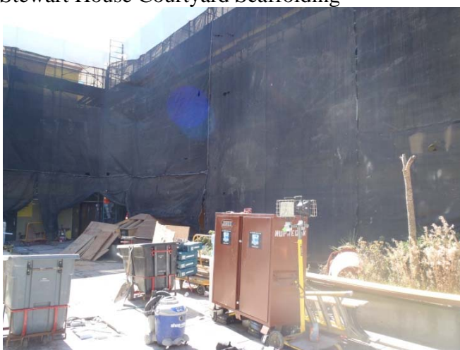
Scaffolding and Protective Netting in Stewart House Courtyard
