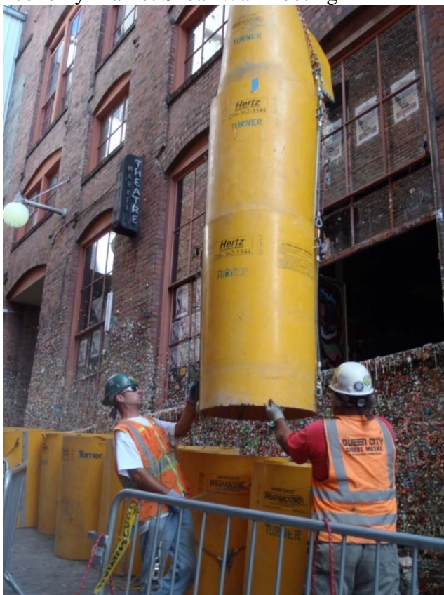
Building a trash chute Economy Market
