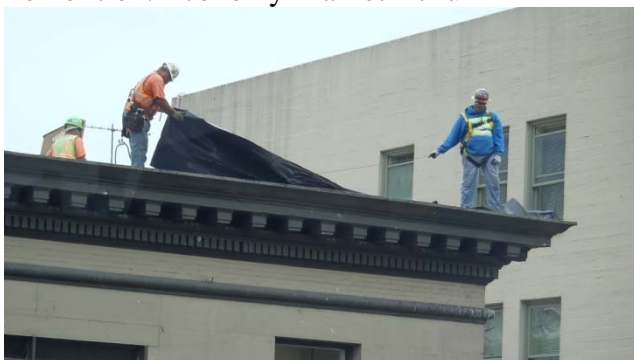
Roof Work: Economy Market
