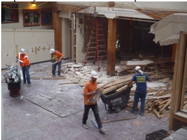
Demolition: Economy Market Atrium
