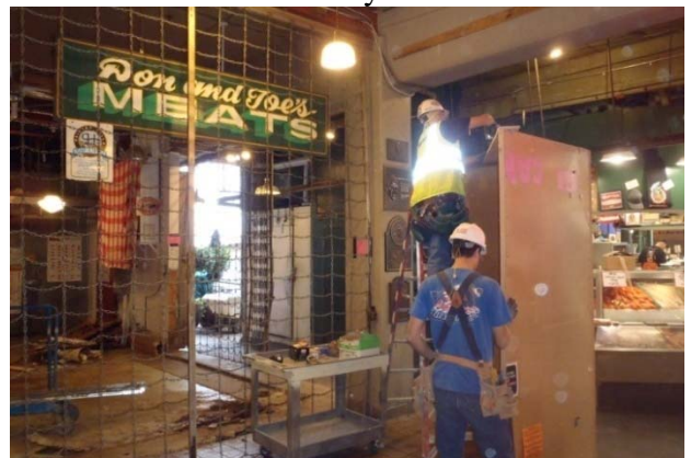
Temp Wall outside Don & Joe's
