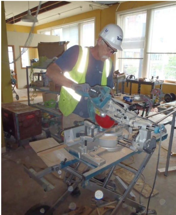
Carpentry Work: Cedar River Group
