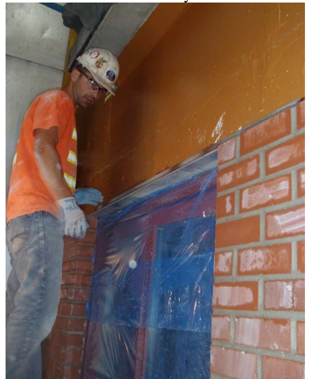
Stewart House Courtyard Window Protection
