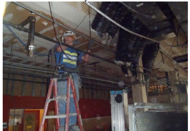
Electrical Work: Economy Market L7
