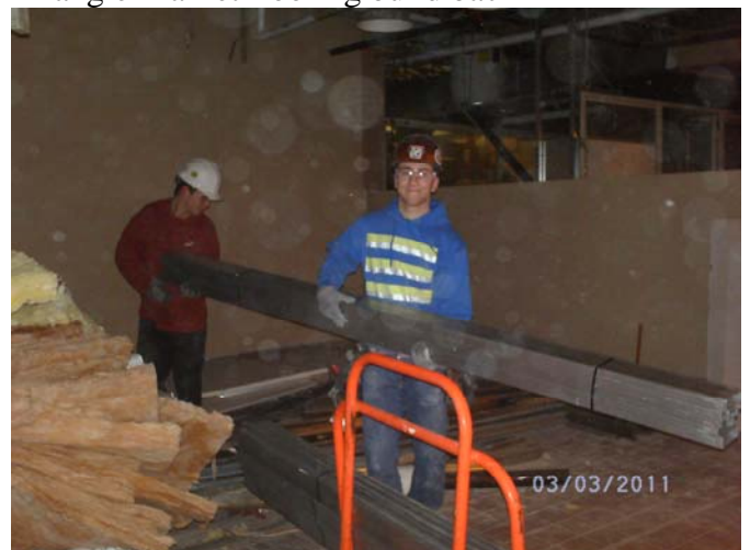
Steel stud framing in Sanitary Market
