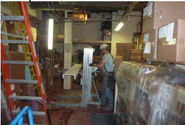
Metsker Maps Drag Strut Installation
