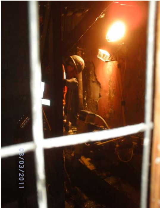
Plumbing Trench near coolers in Sanitary Market
