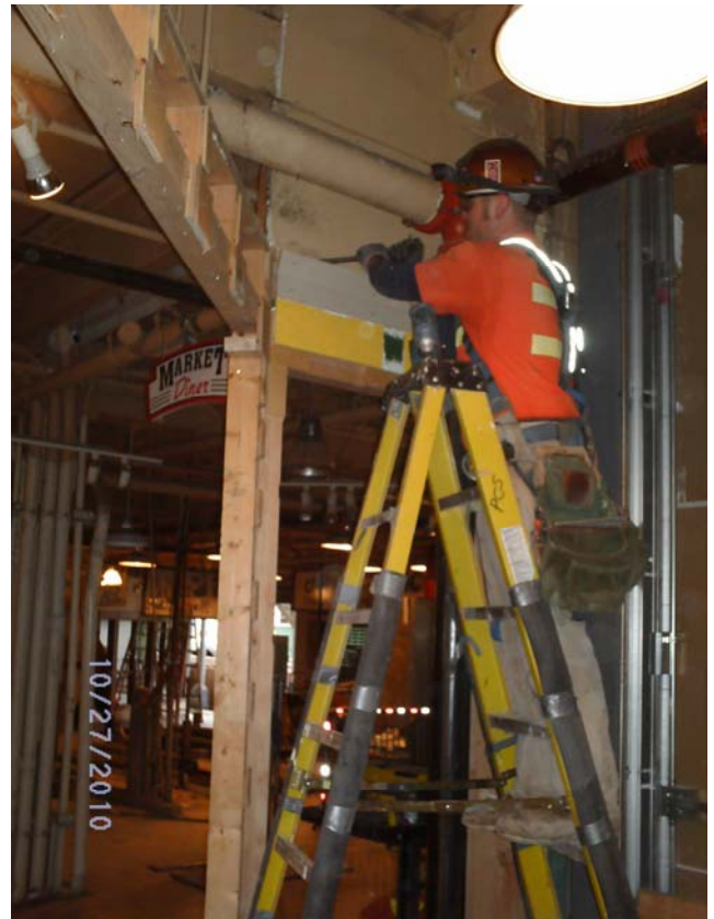
Demolition of wall outside Market Diner
