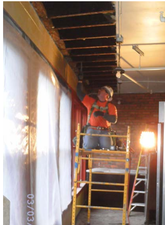
Diaphragm nailing in Copacabana
