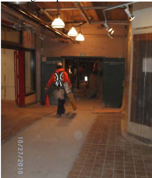
New Concrete over Sanitary Market Trench
