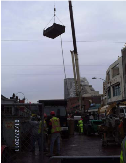
Removing debris by crane from the roof of the Corner Market
