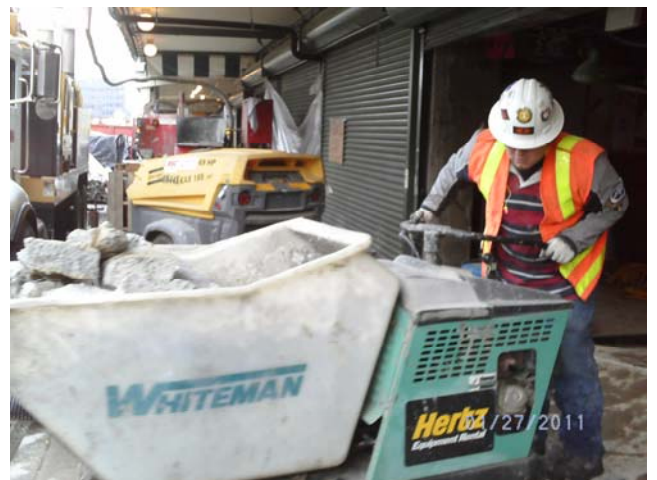
Carting away concrete debris from trenching in Corner Market
