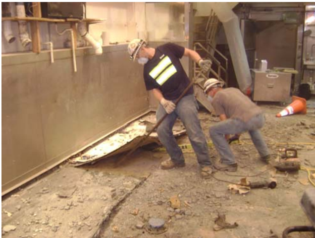
Demolition continues on Pure Food Fish Floor
