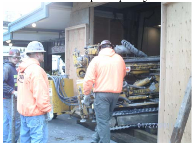
Moving the drill into the Crumpet Shop on First Avenue
