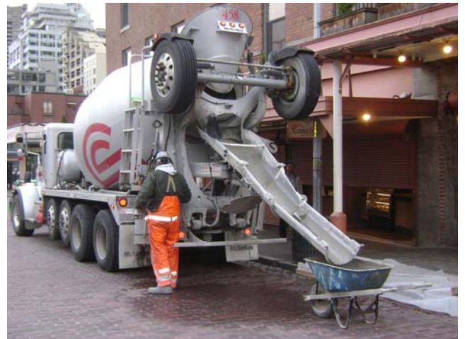
Concrete delivery for Corner Market
