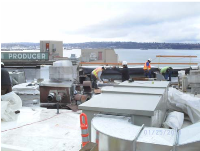
Work on the Corner Market Roof
