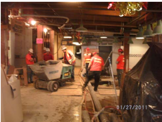
Trenching in the Corner Market
