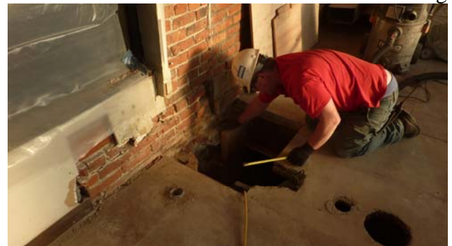
Prepping to Drill for Hombow Brace Frame
