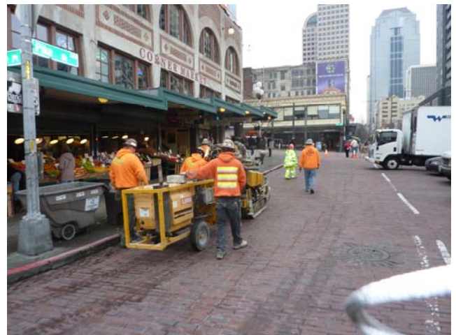
Moving the drill from Corner Market to The Crumpet Shop along Pike Street
