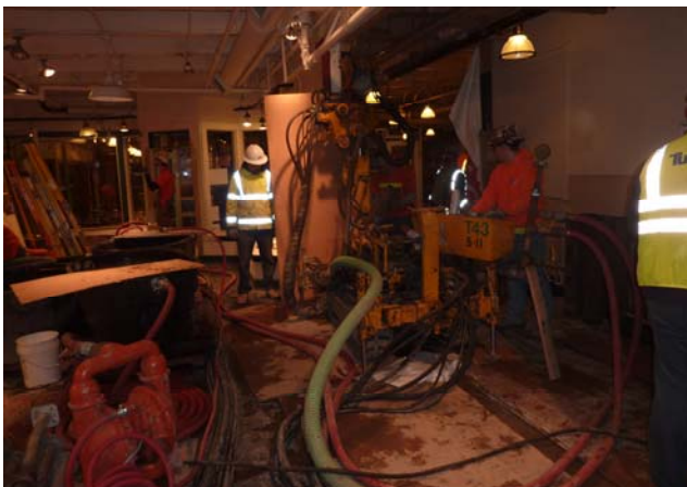
Drilling in Sanitary Market
