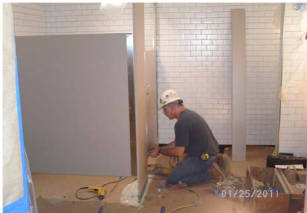
Installing toilet partitions in the Women's Public Restrooms-Sanitary Market
