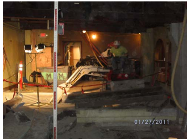
Trenching in tight quarters in Can Can
